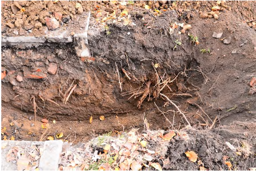
Photo 9 Trial Pit 5 (Under- grass)
