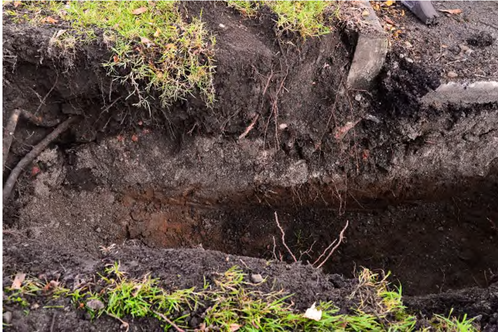
Photo 1 Trial Pit 1 (Under- grass)
