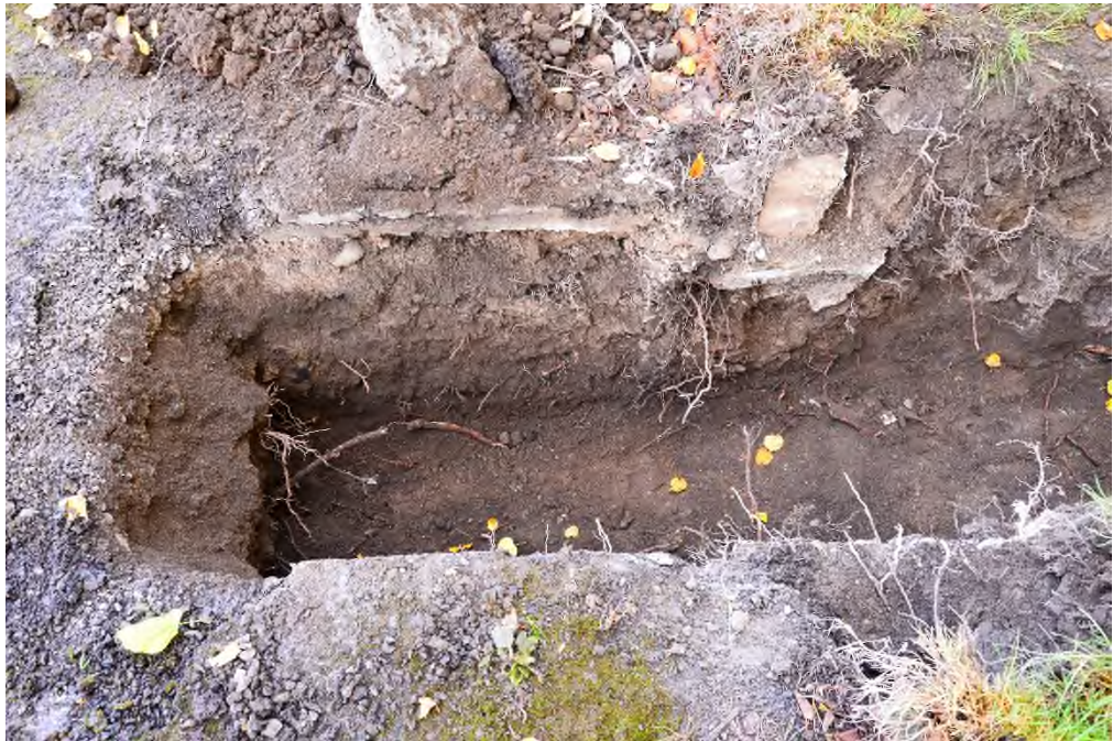
Photo 4 Trial Pit 2 (Under- grass)
