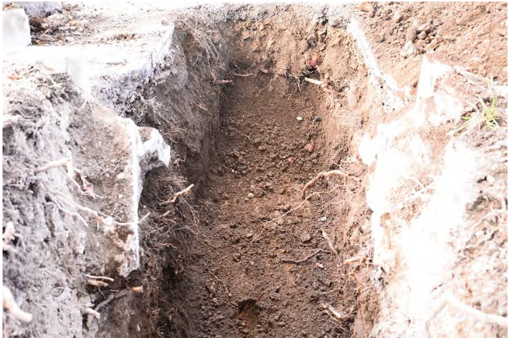
Photo 8 Trial Pit 4 (Under- road)
