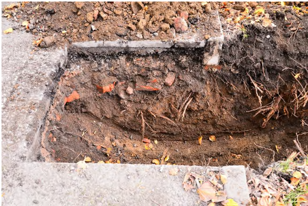
Photo 10 Trial Pit 5 (Under- road)
