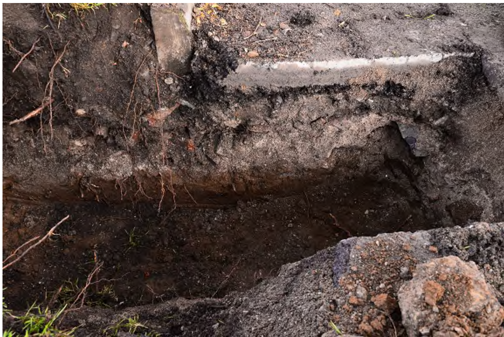
Photo 2 Trial Pit 1 (Under- road)
